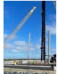
Entergy Texas' Bo Reliability Project phase of construc
